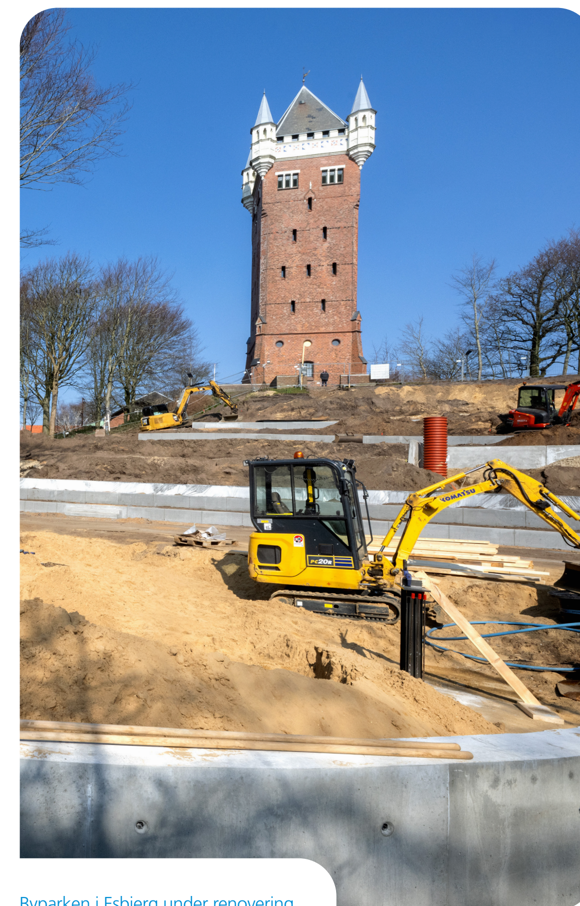
Byparken i Esbjerg under renovering.
